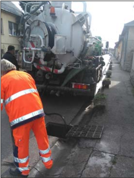
Árpád street - duct cleaning
