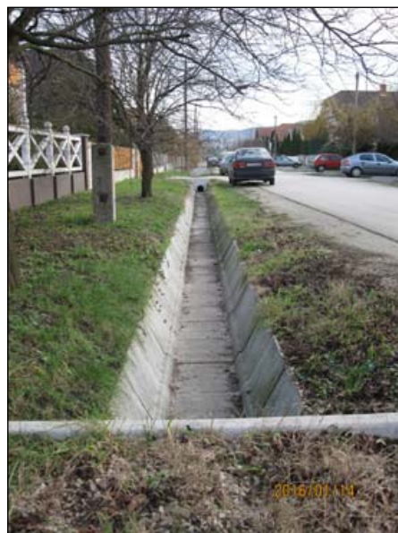
Liszt Ferenc street - ditch cleaning
