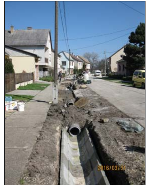
Béke tér - new ditches and culverts
