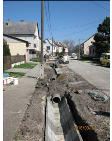
Béke tér - new ditches and culverts
