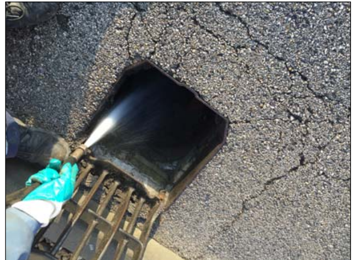
Mogyorósbányai street - duct cleaning
