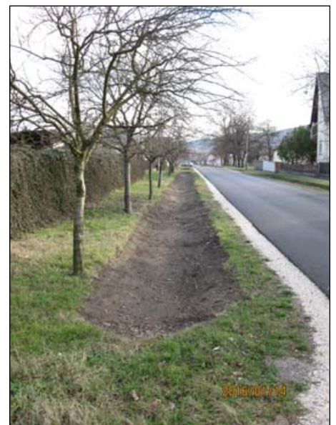
Vak Bottyán u. - ground ditch maintenance
