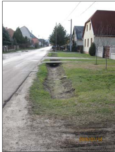
Babits street - ground ditch maintenance
